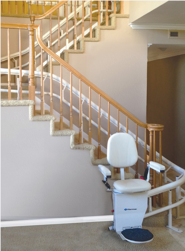
Beige rail with tight 180° turn on the inside wall of stairs
