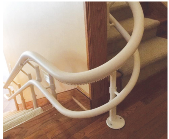
Beige rail with tight 180° turn on the inside wall of stairs
