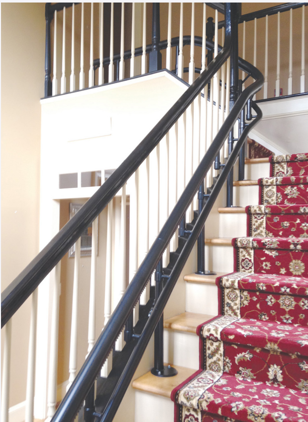
Black rail with 90° turn against the banister side of the stairs
